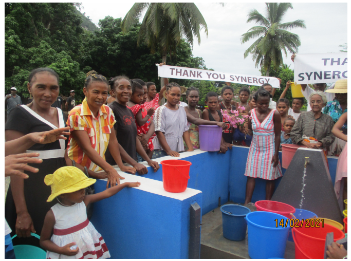
Clean water system in Ambolomadinika
